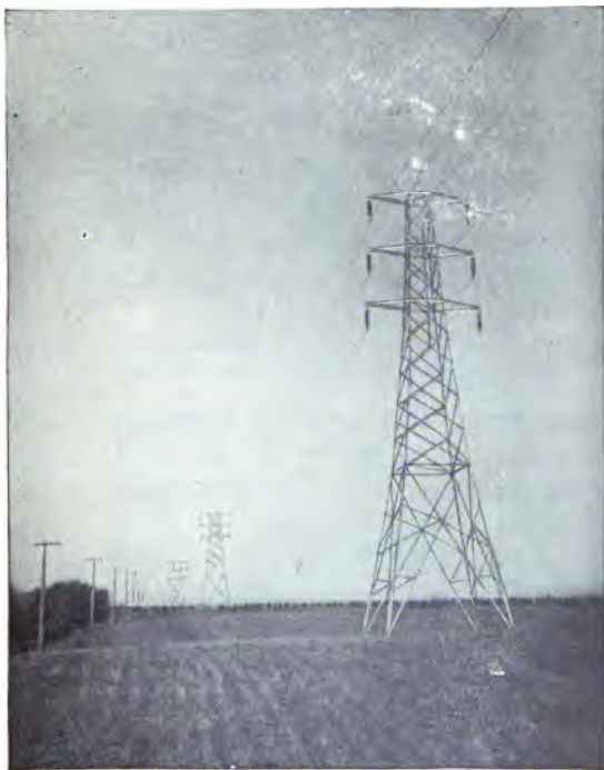
FIG. 221a. A section of the 110,000-volt line from Keokuk, Iowa, to St. Louis, Mo. General Electric Review .
